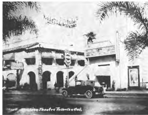
Fox Fullerton Theatre in Fullerton, CA. Photo courtesy of Fullerton Historic Theatre Foundation.
